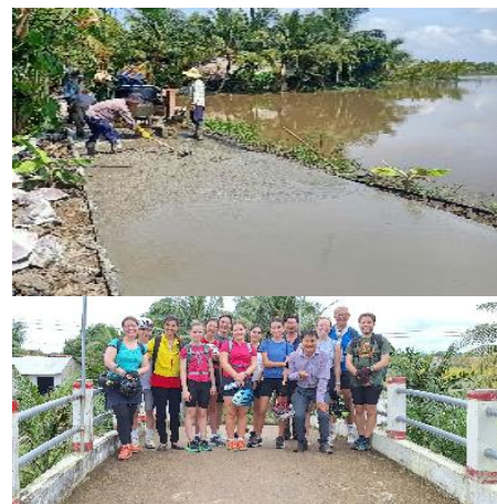
Road and bridge support
